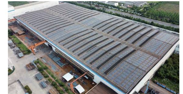
Distributed photovoltaic power generation panel
