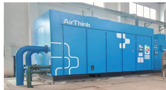
Renovation of the air compressor
